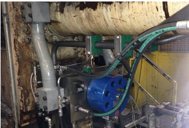
Figure 1 - Operator Side View of Meter-Out Hydraulic Circuit Upgrade.
